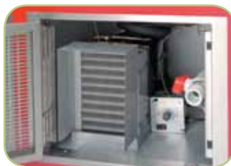
Easy access to temp controls, condenser coil and valves
